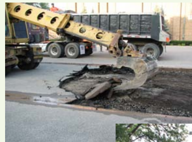
Removing concrete to prepare the bioswale site.
